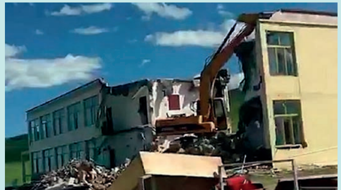
A Tibetan building is torn down near Lake Qinghai.
